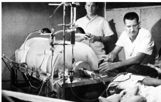
FIGURE 140.1 Early (c. 1950) treatment of acute renal failure using the Kolff-Brigham dialysis system.
